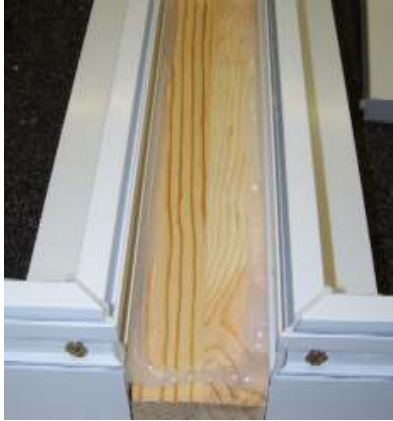
Figure 07. Section Detail of Sealant Location
