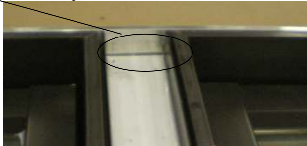
Figure 24. Photo of Sealant Location
