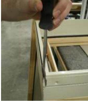
Figure 15. Photo of Notching Method
